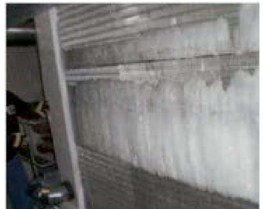
Fig. 3: Iced evaporator.
