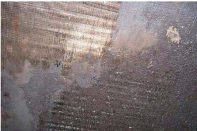
Fig. 1: Soiled condenser; the plate fins close slowly.
